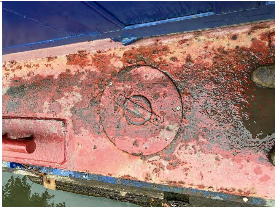
Description: Fuel tank; 2 onboard with ~2,400 gallons total; blueprint ref. V
