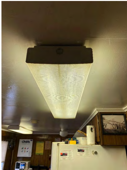
Description: 6 fluorescent tubes and ballasts kitchen; blueprint ref. C
