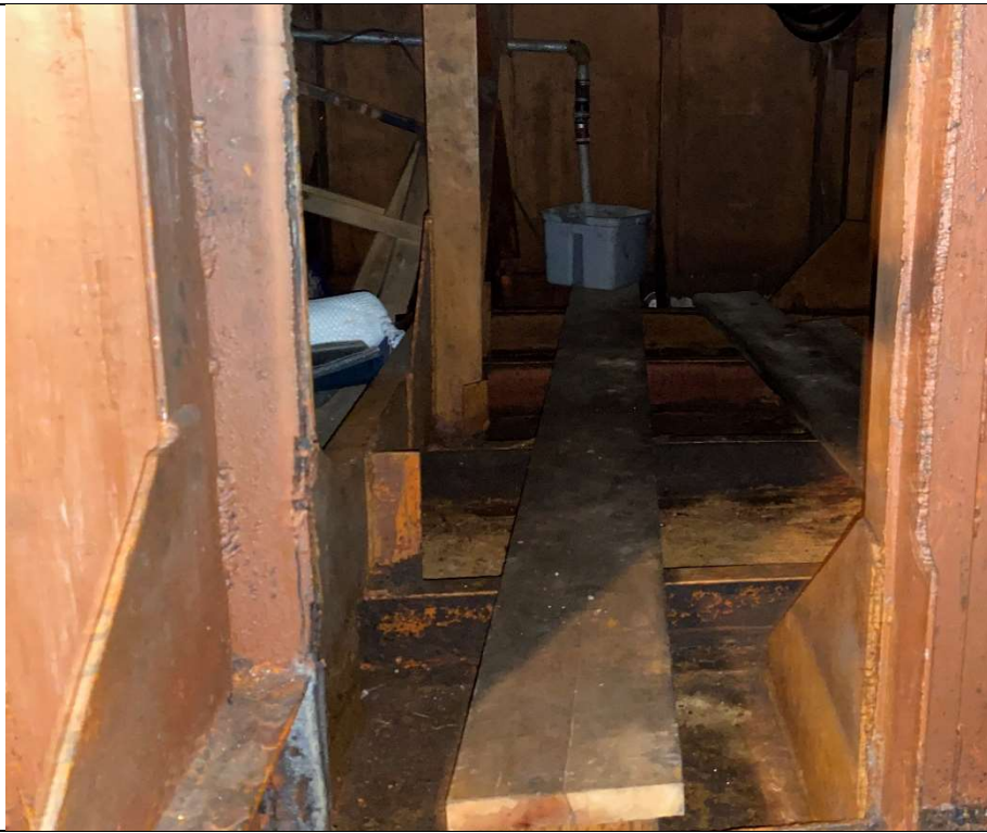
Description: Forward of engine room
