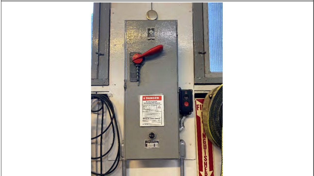
Description: Motor control box; blueprint ref. P
