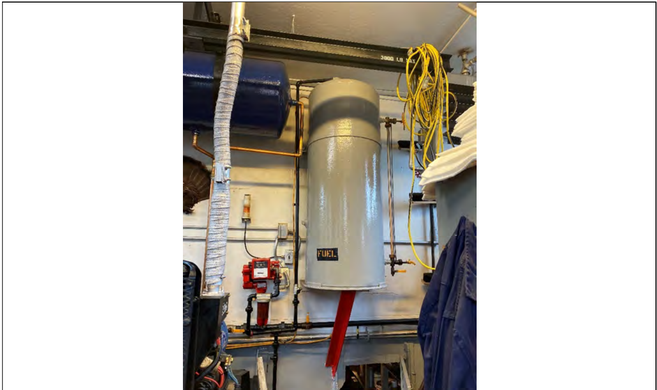
Description: Fuel tank with ~100 gallons diesel fuel; blueprint ref. S
